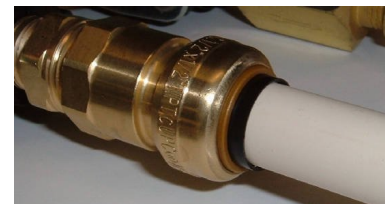
1/2" push fittings supply wall and hand shower piping
