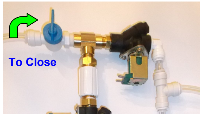
Valve shown in closed position
